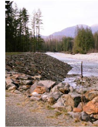
New dyke along the Chehalis River
